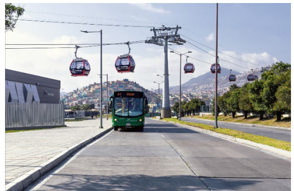
Caption 4: In Bogotá/Colombia, the TransMiCable in the Ciudad Bolívar district closes a gap in the bus network and noticeably reduces road congestion. (Photo: Doppelmayr)
