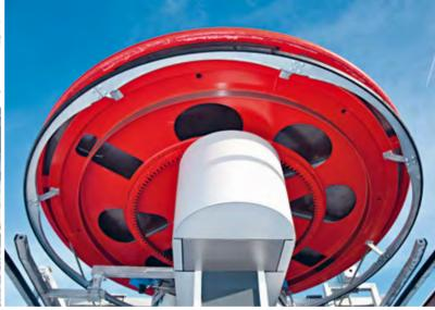
Fixed chairlifts also come with a wide range of drive options. Whether situated in the top or bottom station, the drive can be designed as an underground or overhead version as well as the standard configuration consisting of a compact ChairDrive. The striking features of the ChairDrive are the clear layout of the various components and their compact construction, which make installation and transport very straightforward and efficient.
