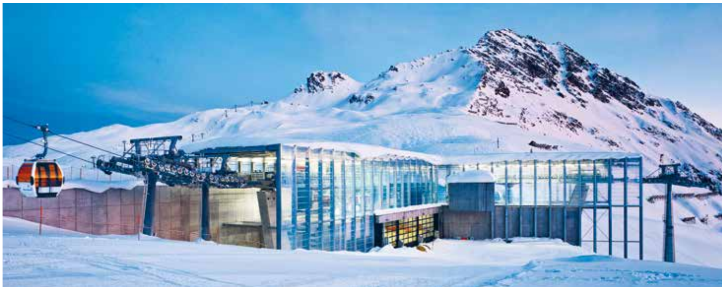
The Grasjochbahn (AUT) is the first detachable gondola lift where Doppelmayr implemented its innovative recovery concept.
