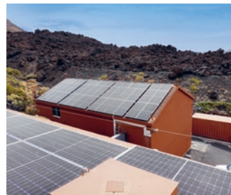
The Pico del Teide aerial tramway generates carbon-neutral energy with PV installations on all building roofs. The ESFOR system is used to store the energy.
