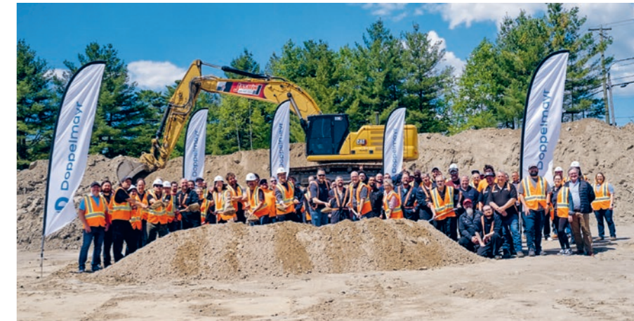
In a small celebration, Doppelmayr Canada marked the groundbreaking for the new building in Saint-Jérôme.
