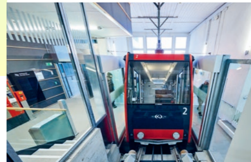
The Leubringen funicular in Biel is fully automated, and the vehicles and stations comply with the requirements of Switzerland's Disability Discrimination Act.
