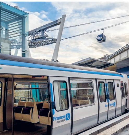
Conventional forms of mobility at street level are reaching their capacity limits in metropolitan areas. Ropeways take urban mobility to a new level.
